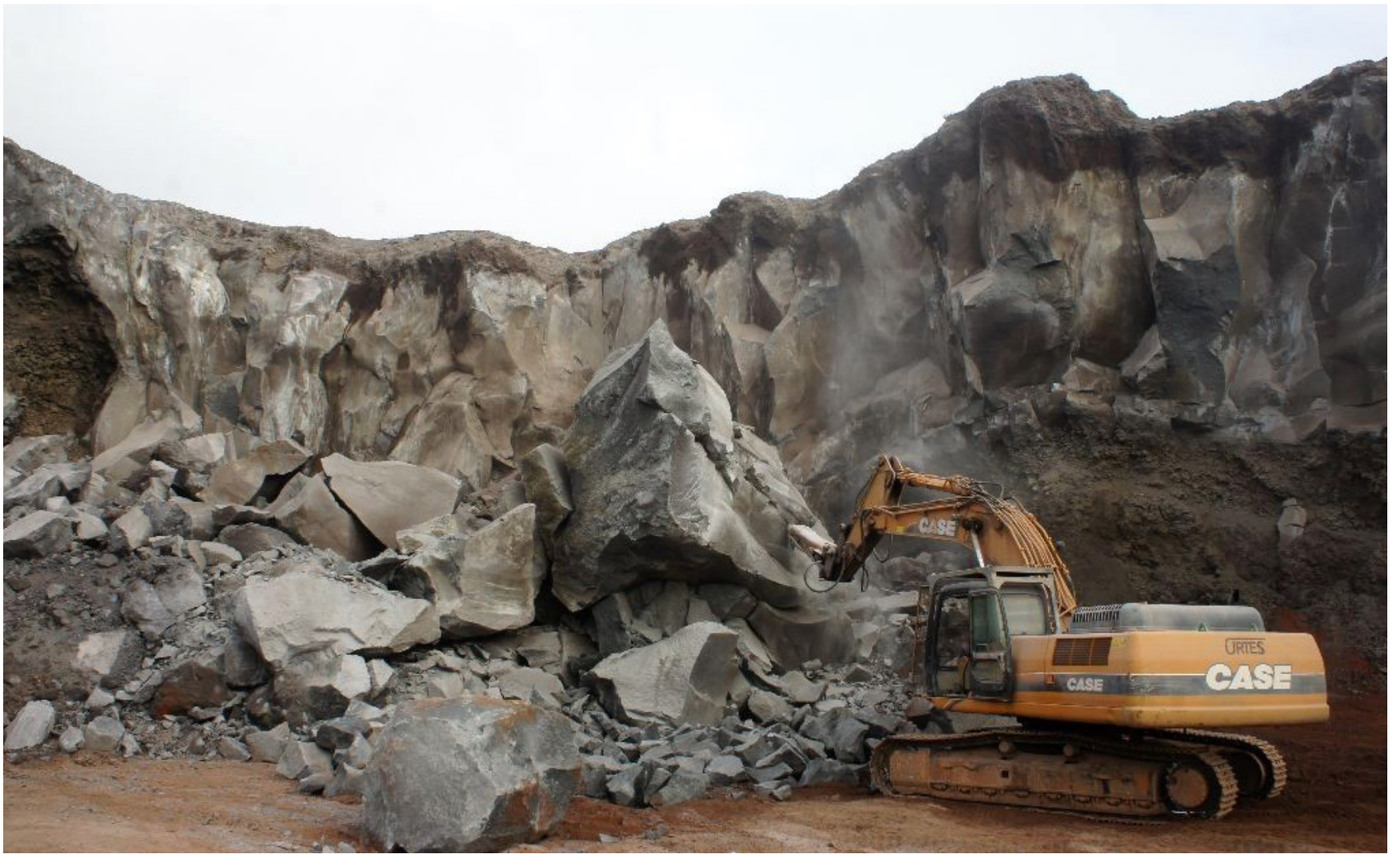
Extraction by underdigging
