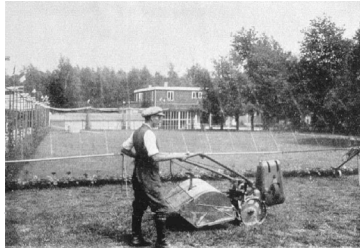
4. This larger-scale garden was intended for settlers who derived their primary income from their garden. Migge embraced the use of technological devices such as the new electric tiller. In the background is a house with a window palisade. Reproduced from: Leberecht Migge, Deutsche Binnen-Kolonisation , p. 71.
