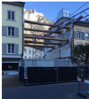
Construction props
