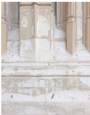
Repaired stone facade
