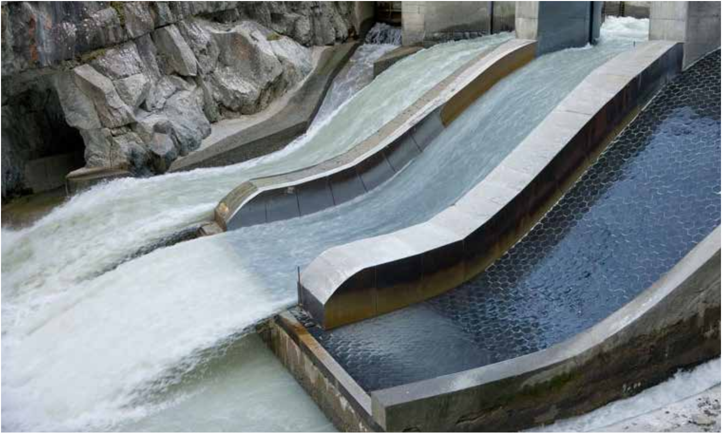
MOREL HYDROPOWER PLANT
