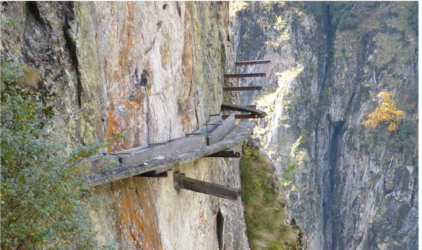
(FORMER) BISSE DE RIEDERI (water channels)
