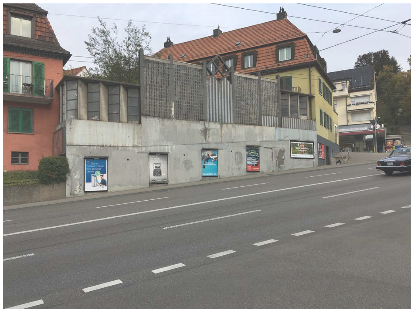
Closed Courtyard along the Rosengartenstrasse, 2021
