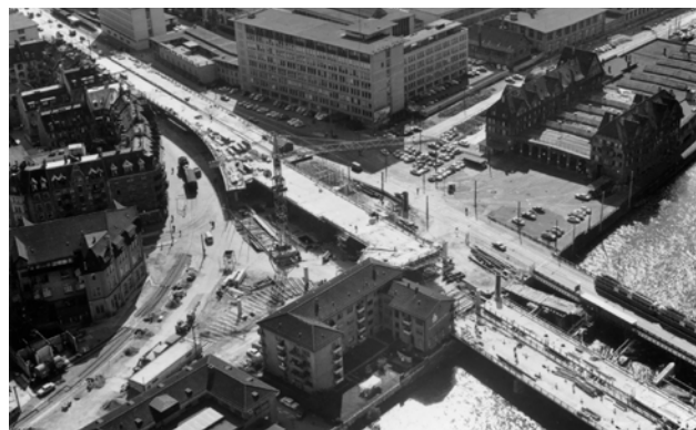
Wipkinger bridge and Eyscherwyssplatz covering under construction, 1969
