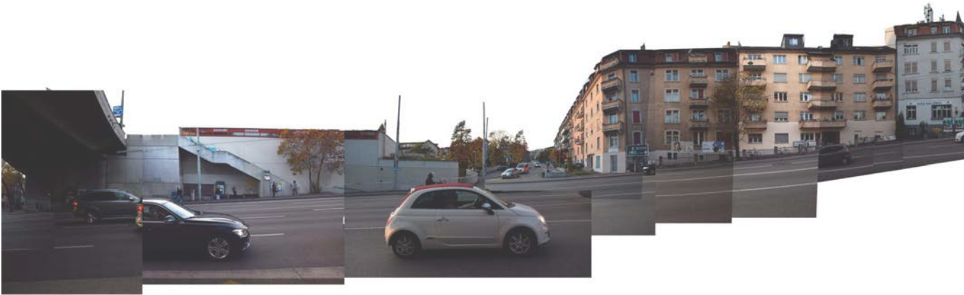
Pedestrian Bridge - Front View Collage
