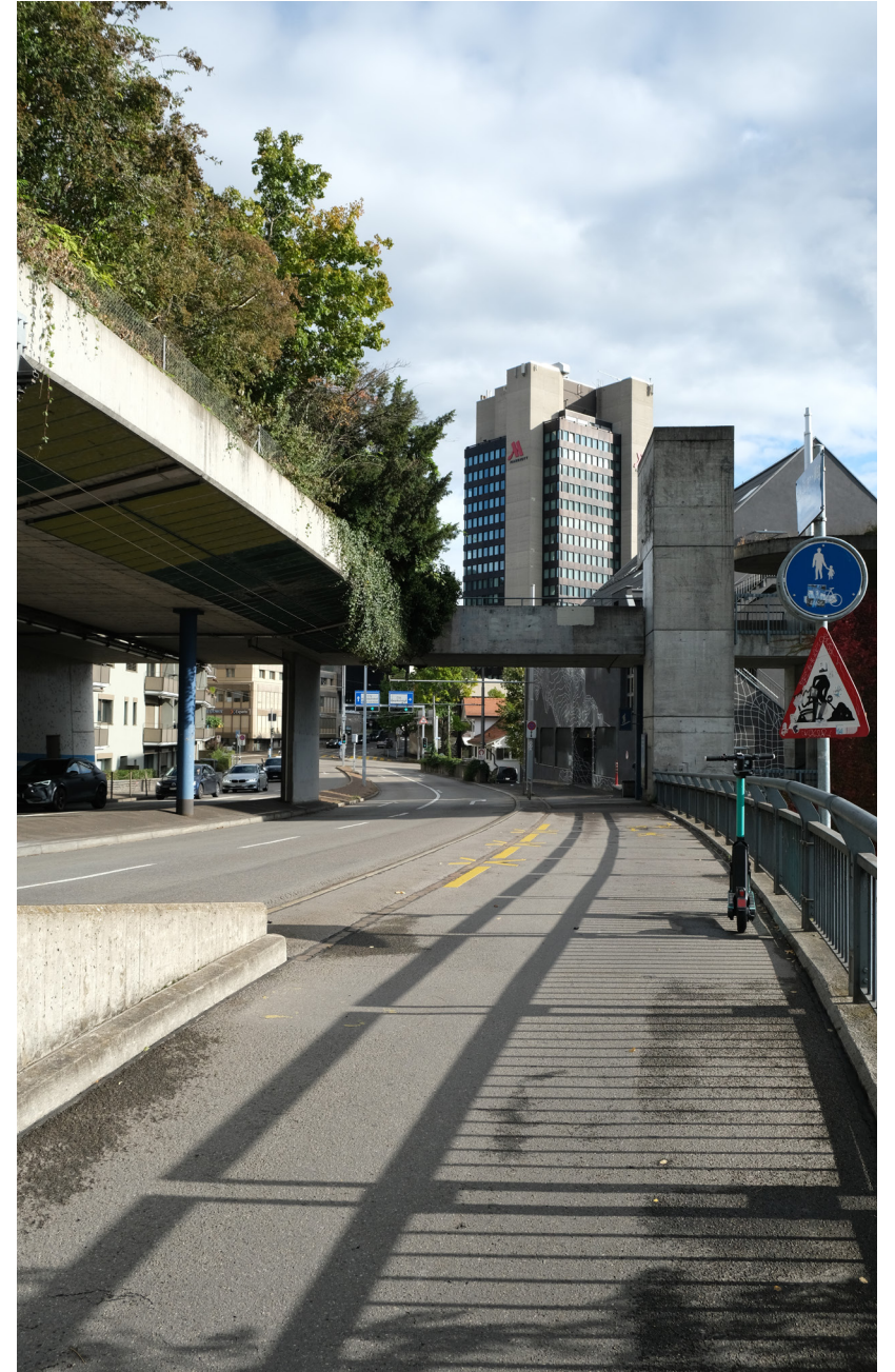
pedestrian link between Dynamo und Schigu
