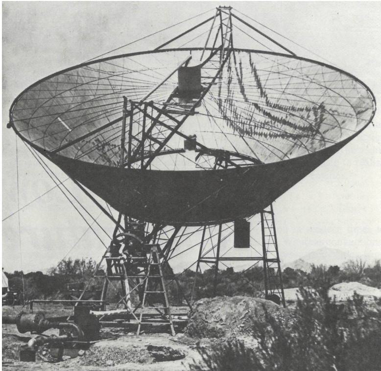
1900 AUBREY ENEAS SOLAR MOTOR WITH CLOCK MECHANISM ROTATING THE MIRROR ALONG A TOWER
