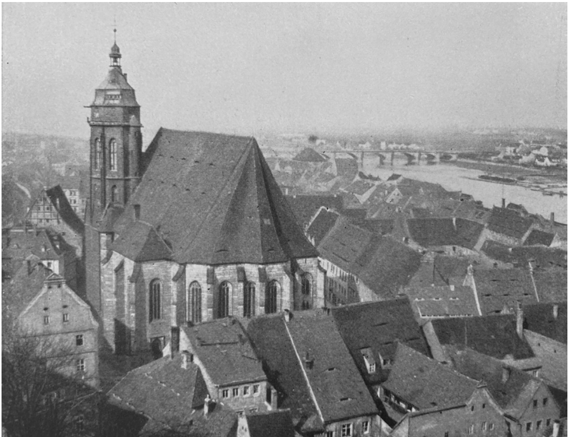
Harmoniously integrated church complex.
