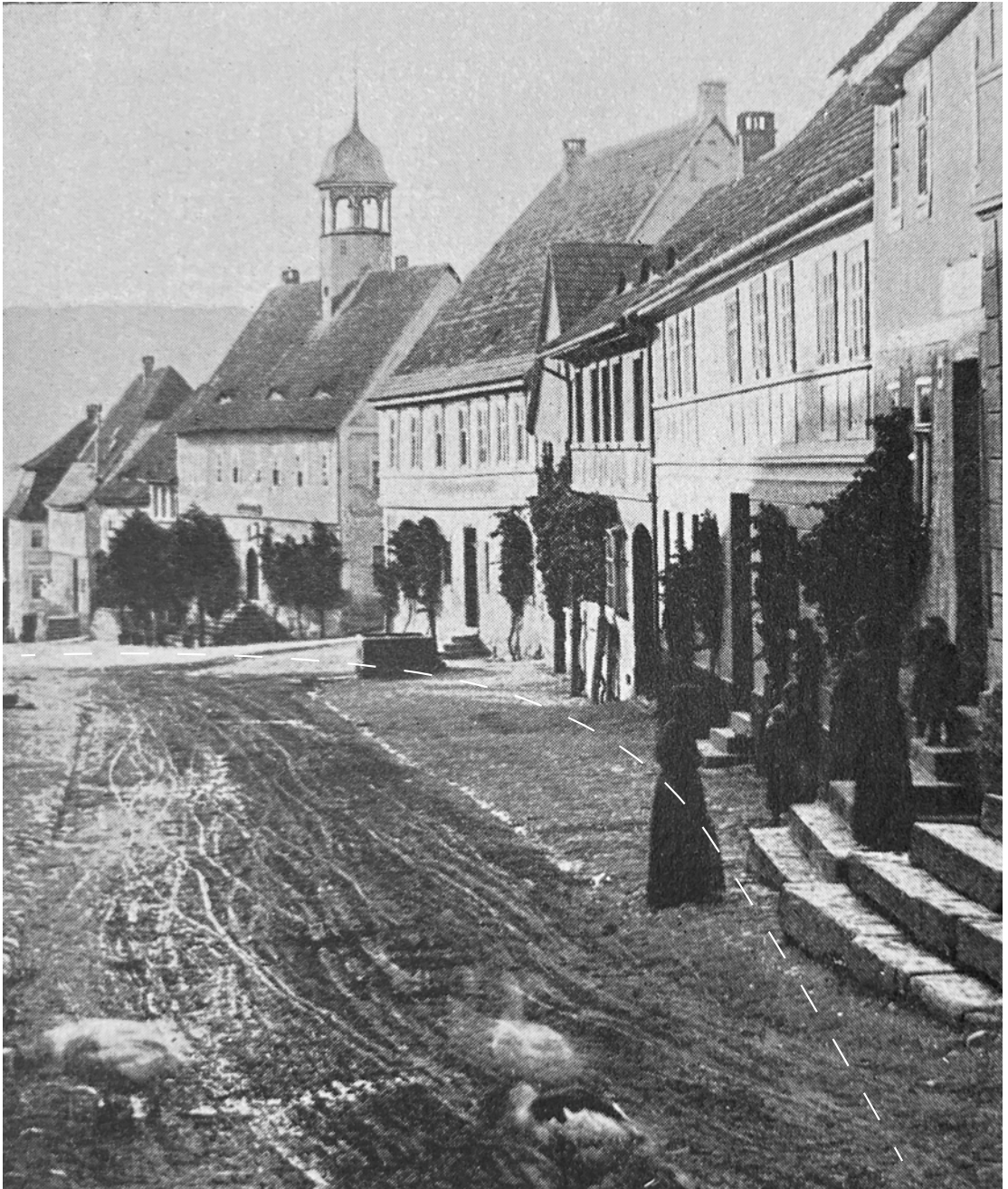
The good curvature in a street alignment makes all house fronts visible.
