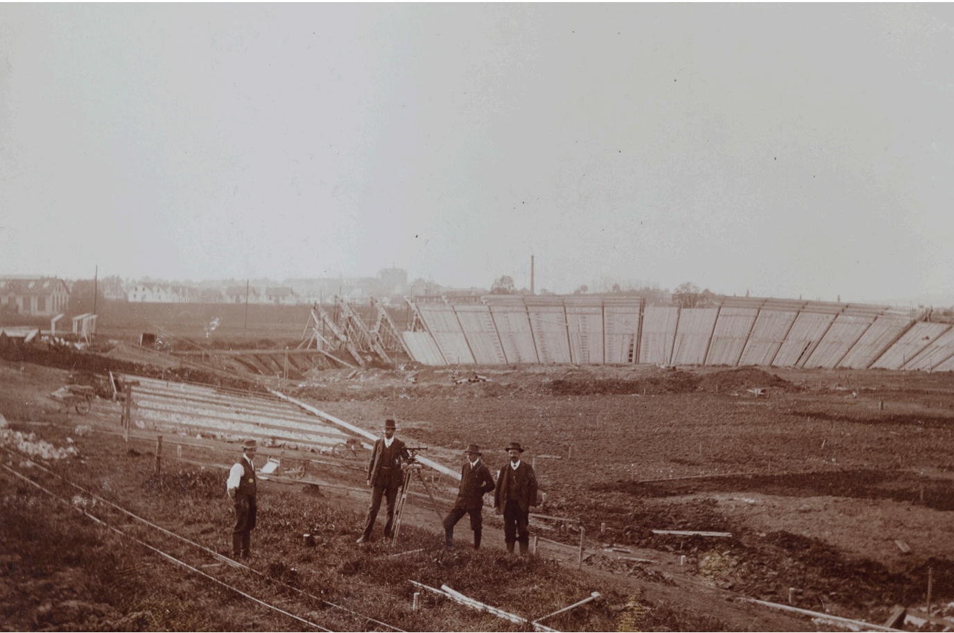
Construction of the racetrack, 1912. Baugeschichtliches Archiv, BAZ_168601
