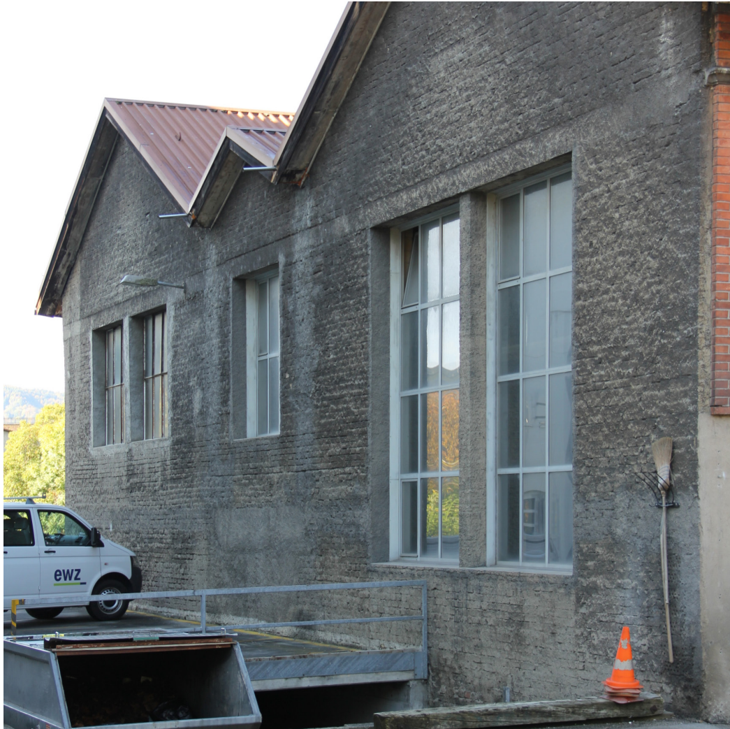
wall of detached part
