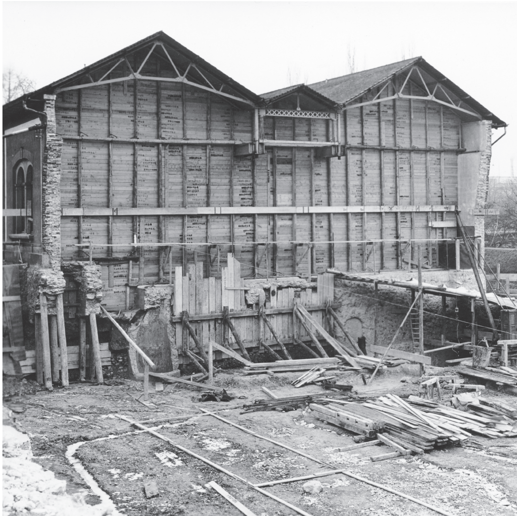
split: destruction for construction of Unterwerk
