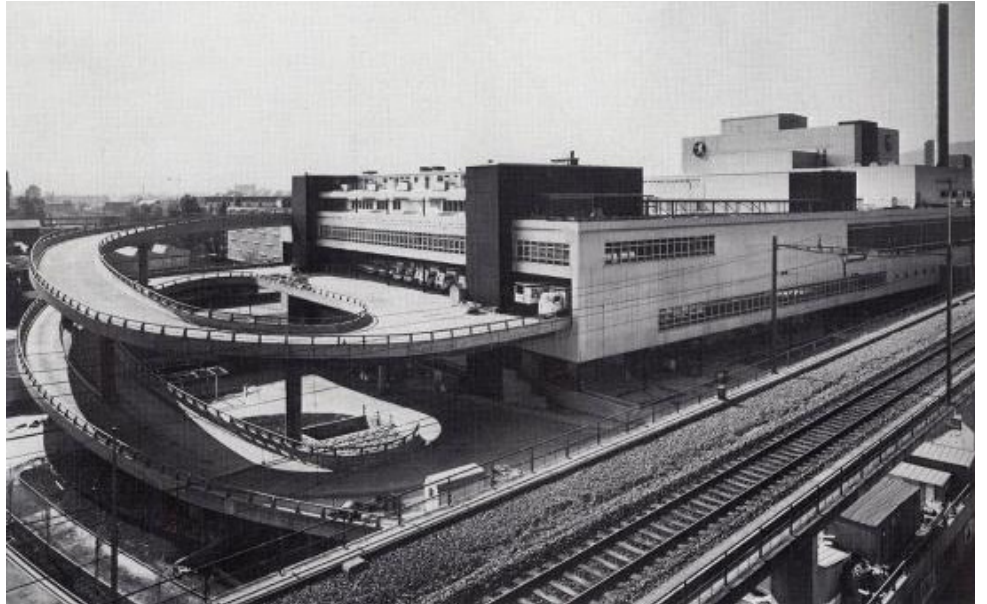
Toni-Molkerei, Nord-West Fassade (2007)
