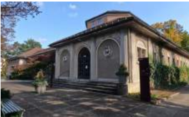
Figure 79: New Mortuary Exterior. by Author. (2022). [img]
