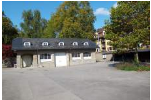
Figure 87: Equipment Storage Building. by Author (2022). [img]
