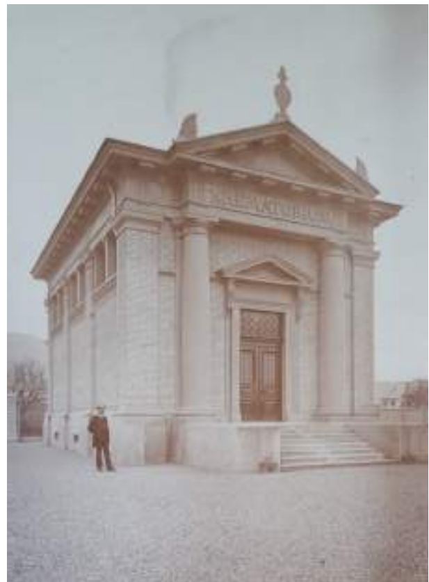
Figure 63: Old Crematory exterior photo. Archive Stadt Zurich (1877). [img]
