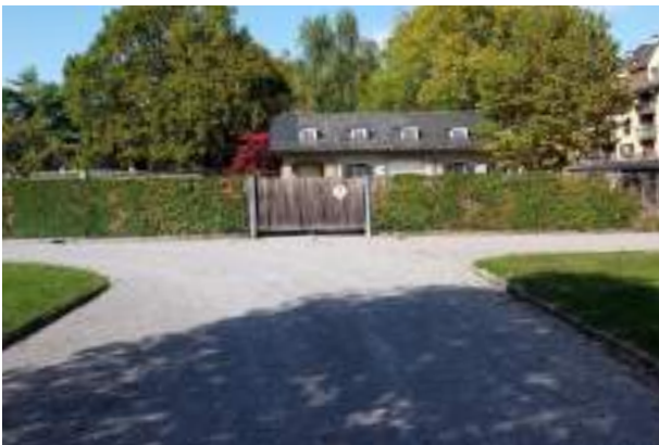
Figure 86: Equipment Storage Building, gate view from inside Sihlfeld A. by Author (2022). [img]
