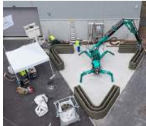
Figure II5: Construction 3d Maxi Printer. Source: https://en.constructions-3d.com/la-maxi-printer . [image]
