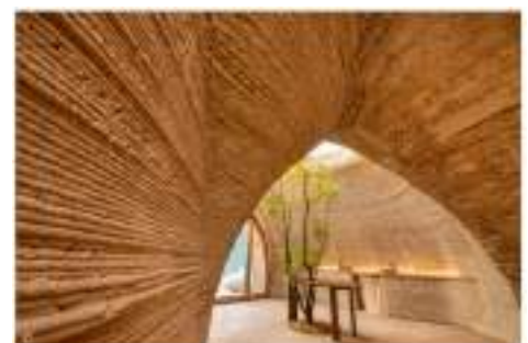
Figure II6: 3d Printed clay house, Tecla, by architect Mario Cucinella. Source: https://www.archdaily.com/960714/tecla-technology-and-clay-3d-printed-house-mario-cucinella-architects . Image by: Iago Corazza. [image]
