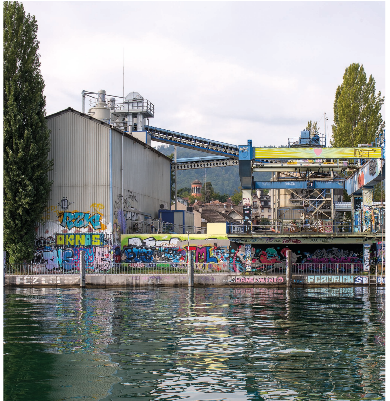
Concrete Plant Zurich- Wollishofen Kibag Image: Haller, Juliet, BAZ, 2021.
