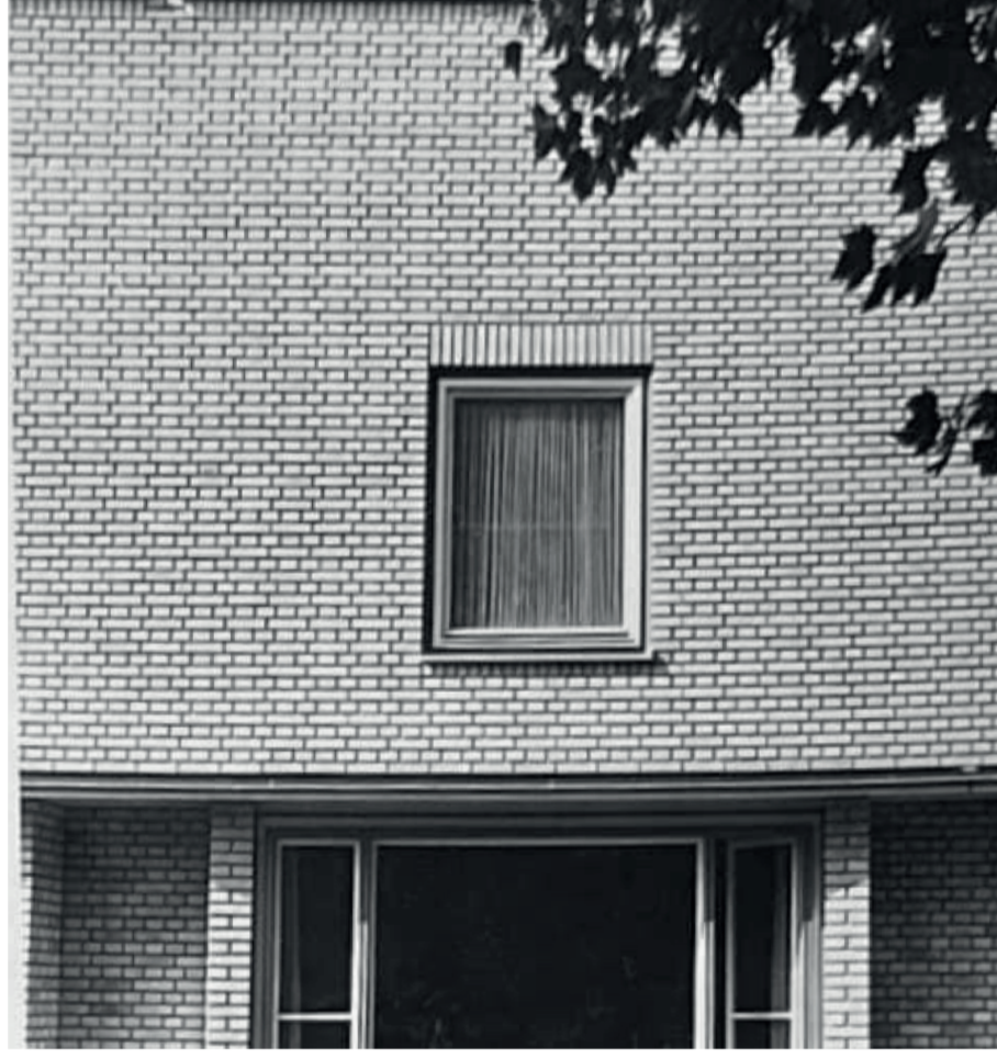
Kantine Escherwyss, Zurich Completion of the brick facade up to the roof and window lintel. Reference for the window lintel and facade termination.
