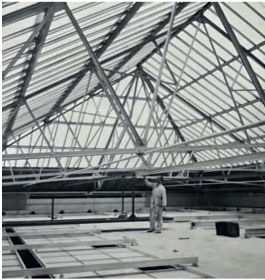
Sammlung Oskar Reinhart am Römerholz, Winterthur Transparent roof for indirect light of the exhibitions rooms underneath. Reference for the roof and the Whit box exhibition rooms.
