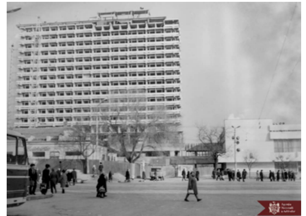
Image of the construction process of the hotel, the last floors being erected. The restaurant building on the right is already finished and functioning. The small houses in front on the left side will get demolished the moment the construction works for the square start, around 1974 (source: Agenția Națională a Arhivelor)
