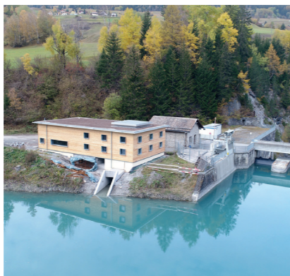
power plant Adont
