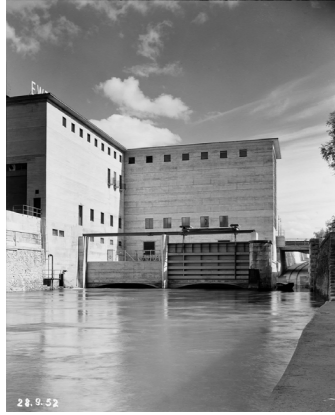
power plant Letten
