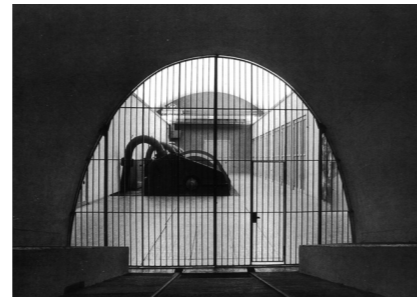
power plant Castasegna
