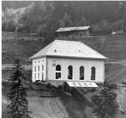
power plant Solis
