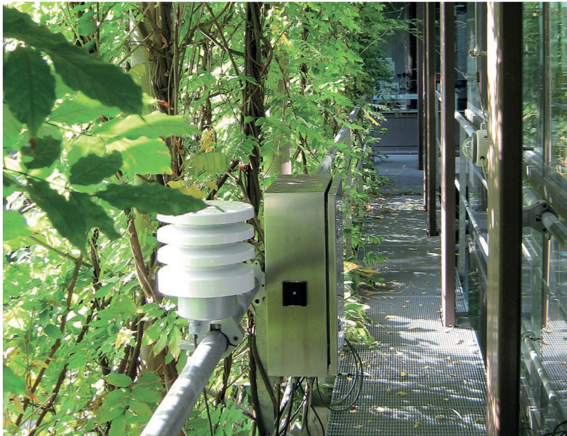
Rainwater irrigation facades examples as string element of the building
