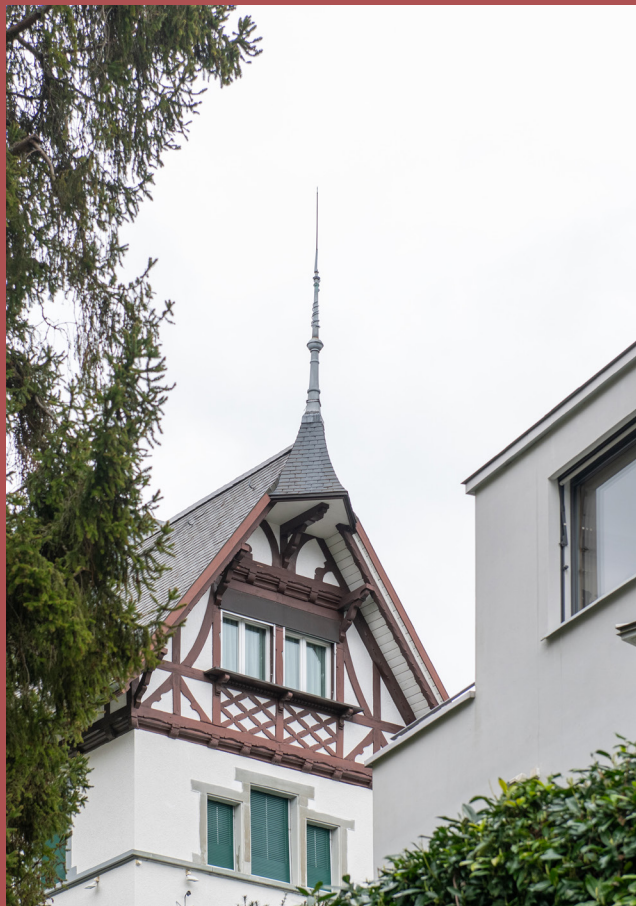
The roof spire of a villa at Kurhausstrasse 10.
