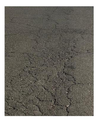
Temperature fluctuations (hot and cold cycles) lead to thermal aging, where repeated expansion and contraction of asphalt occur. In extremely hot conditions, asphalt softens and deforms (rutting), while in cold conditions, it becomes brittle and cracks. Over time, this continuous thermal stress can significantly degrade the pavement's structural integrity.
