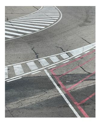
Chemical reactions within the asphalt binder can cause it to harden or break down. This can be influenced by the presence of contaminants like fuel spills, deicing chemicals, or acid rain, which can degrade the bitumen and accelerate aging.
