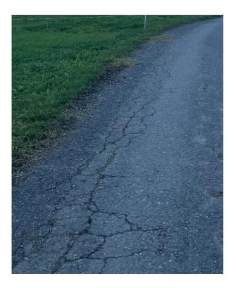
Asphalt pavements experience mechanical aging due to continuous exposure to traffic. The repetitive stresses from vehicles cause permanent deformations (like rutting) and cracks over time. While high-quality asphalt can resist such stresses initially, mechanical aging eventually leads to fatigue cracking and surface wear.
