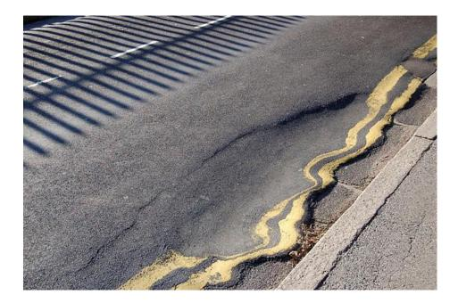
Asphalt is temperature-sensitive: it softens in extremely hot weather and becomes brittle in cold weather. In high temperatures (40°C-70°C), the bitumen can become too pliable, causing the asphalt to rut or deform under heavy traffic. Conversely, in cold conditions, it can become more rigid and prone to cracking. This behavior is mitigated by adjusting the mix design for specific climates or by adding modifiers to improve the temperature resistance of the asphalt.
