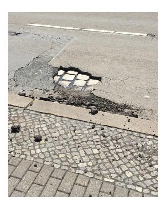
Water penetration accelerates the aging process in asphalt, particularly through stripping, where the bond between bitumen and aggregate weakens due to moisture. The presence of water can lead to potholes, cracks, and other forms of distress, especially if the asphalt is not properly sealed or if drainage is poor.
