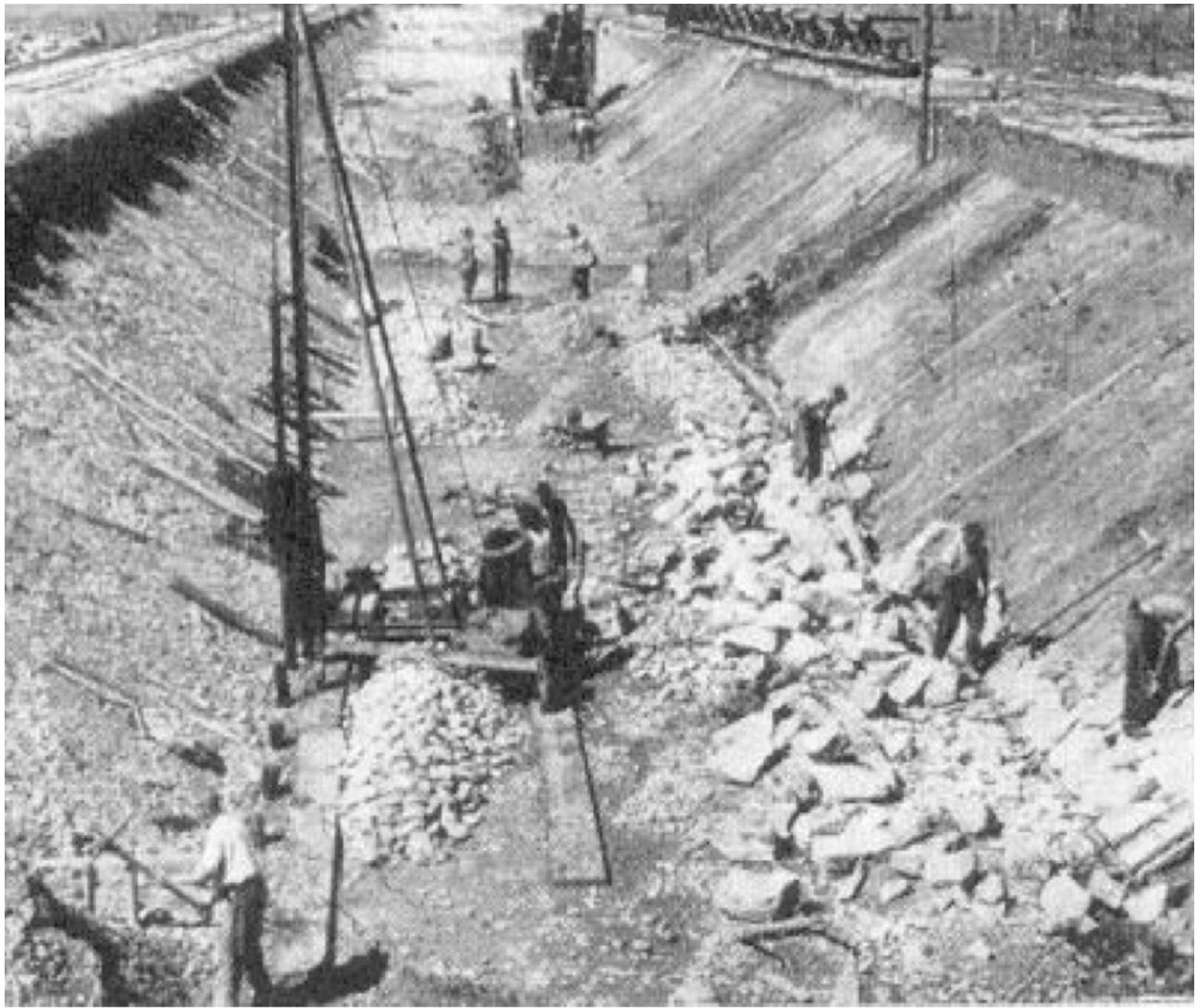
Placing of Slope Paving, 1933
