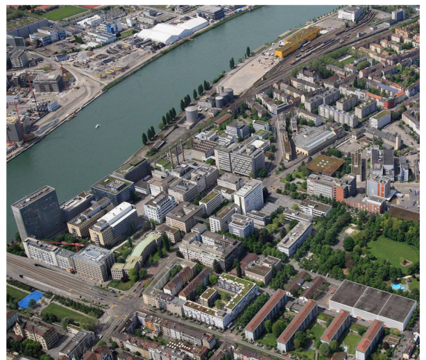
3. Aerial photo of Klybeck Quartier of the campus Novartis
