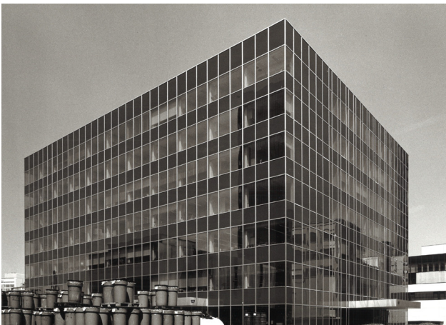
Bau 127 From the South Side
