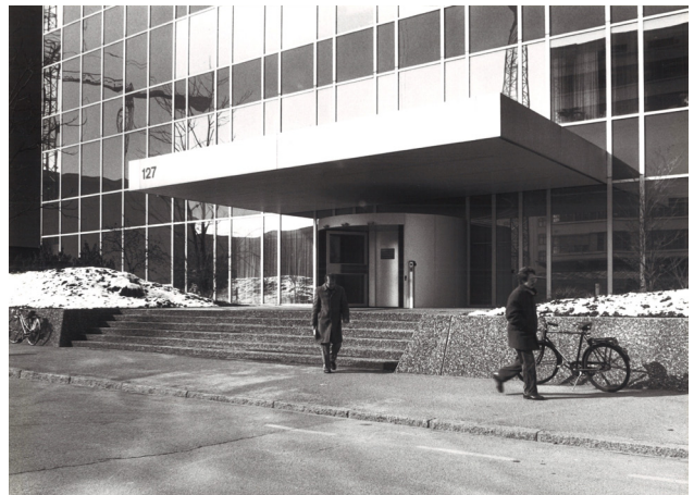
The Entrance Area of Bau 127
